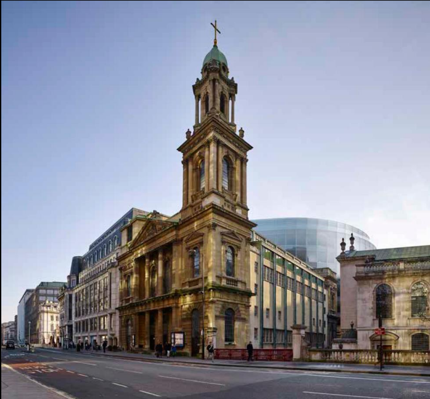
Existing view from Shoe Lane
